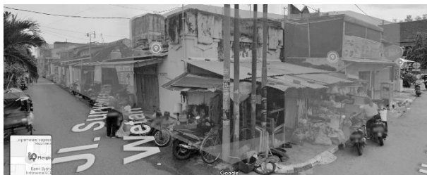
Fig 45. Infilled building (blue) in the ruin of Plengkung Madyasura (red) Source: Google Street view, 2021
