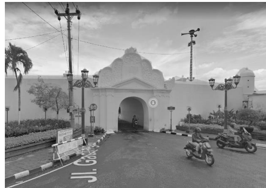
Fig 40. Plengkung Nirbaya now Source: Google Street View, 2021
