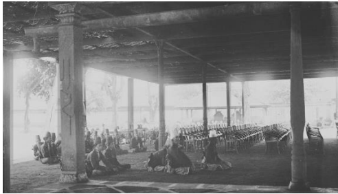
Fig 14. Sitinggil before renovation. Source: (Cephas, 1888)
