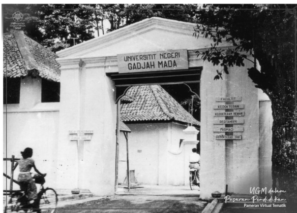
Fig 26. Faculty of Medicine at Dalem Mangkubumen Complex in the 1950s. Source: Khazanah Arsip UGM.
