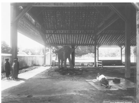
Fig 30. Bangsal Gajahan before renovation. Source: (Kurkdjian, n.d.)
