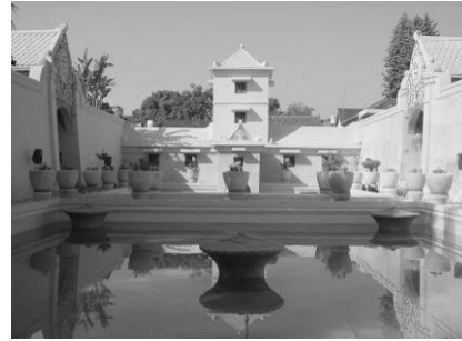
Fig 33. Tamansari after restoration Source: Courtesy of Adishakti, 2005
