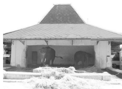
Fig 31. Bangsal Gajahan after renovation Source: Courtesy of Sistem Informasi Nama Rupa Bumi https://sinar.big.go.id/
