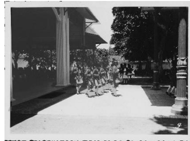
Fig 15. Sitinggil after renovation Source: (Zindler, circa 1930)
