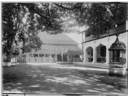
Fig 16. Gedhong Jene before renovation. Source: (Cephas, 1896)
