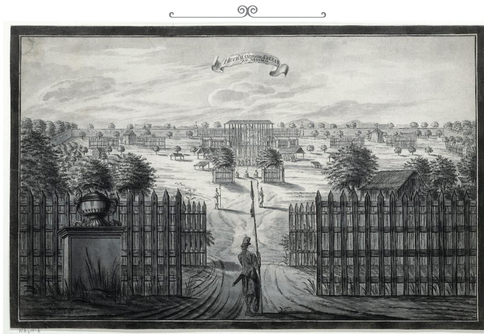
Figure 1. Yogyakarta Royal Palace and Baluwarti Fort Source: Nelly, 1771
